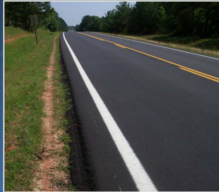
Safety Edge Installation: Georgia
